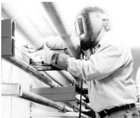
Repairing one of the 4,000 welds in the LCW system.
