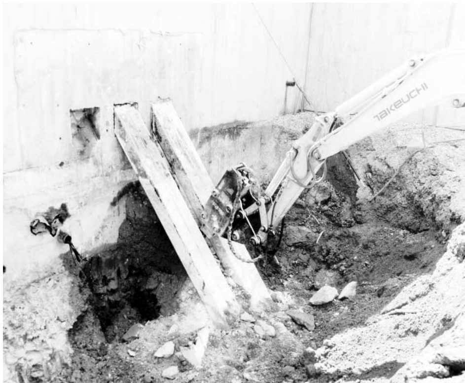
Below the building, 1,450 tons of steel will be inserted as shielding.
