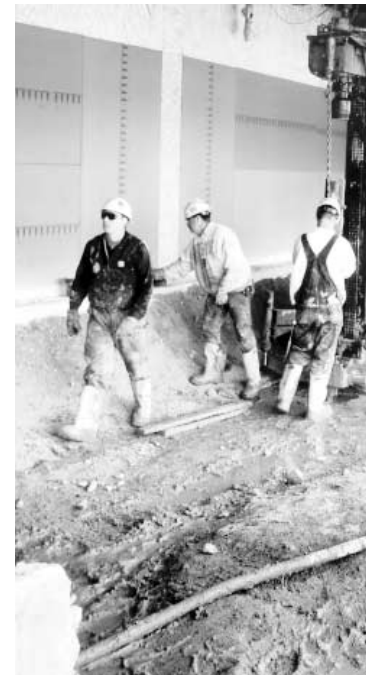
Workers deal with mud at every stage of the Booster shielding project. The building’s beam supports will be carried on “stilts” that are sunk down to bedrock.
