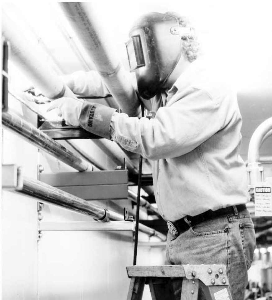
Under contract, workers repaired 4,000 welds in the LCW system.
