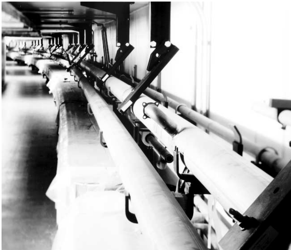
Purchases for the Main Injector included every item inside the tunnel, from magnets to clamps, water systems to light bulbs.
