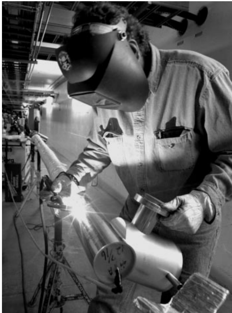
Reed Dewey, of contractor Borg Mechanical, welds sections of the Recycler vacuum tube.
