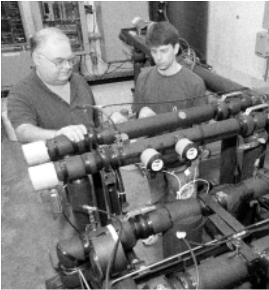
Fermilab physicist Bill Cooper and engineer Dan Olis with the chiller that keeps DZero's silicon vertex detector at -10^{\circ}\text{C} .
