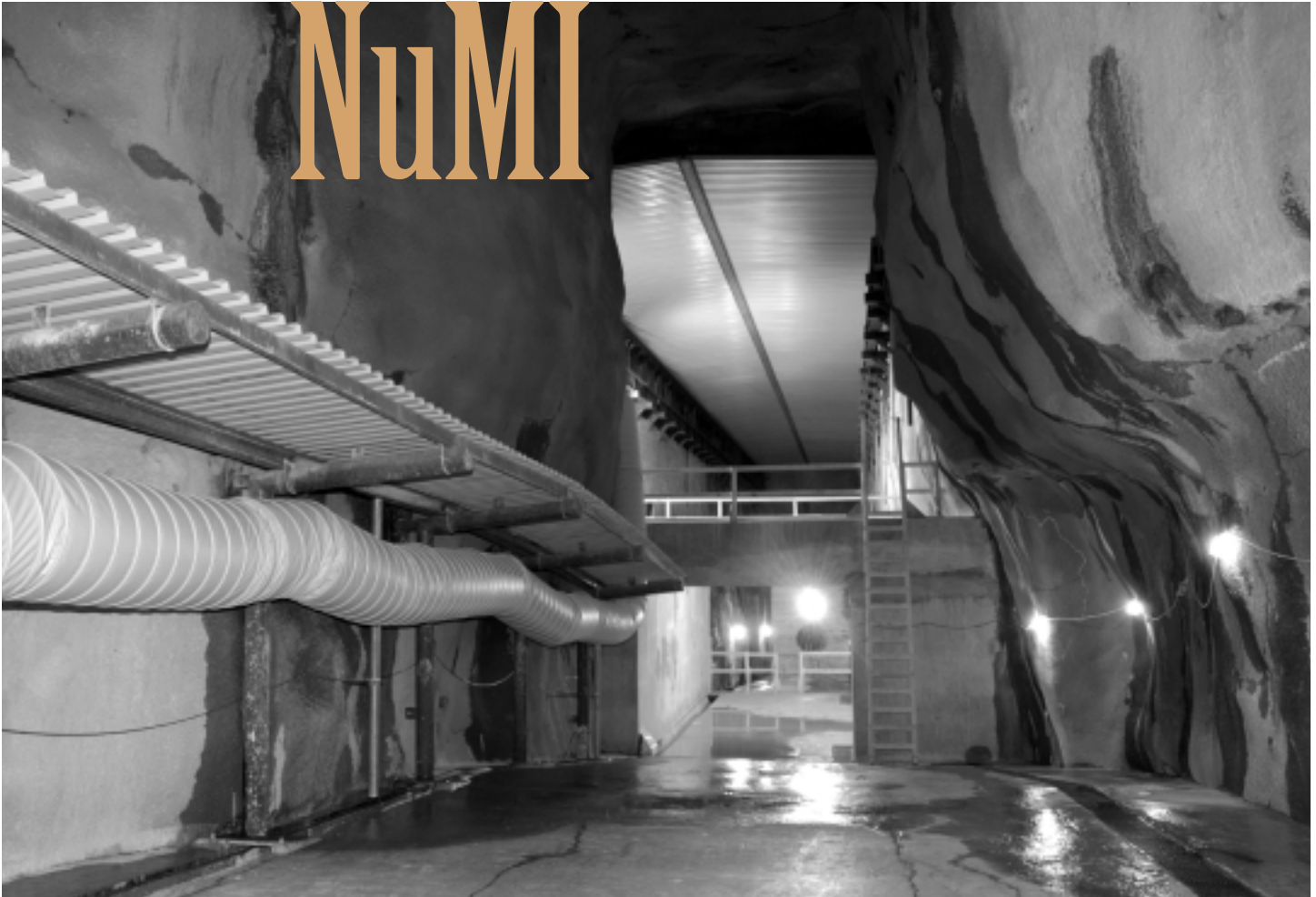
In 2005, a beam line will bring high-energy protons into the 60 foot-high NuMI target hall, where they will collide with a graphite target and create neutrinos.
