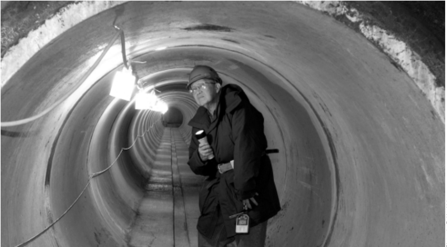
The NuMI carrier tunnel, here inspected by Tony Ramos, will host the beam line that transports protons from Fermilab's Main Injector accelerator to the NuMI target hall.
