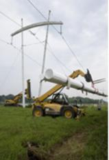
The replacement process of Fermilab's pishaped power lines began yesterday afternoon with the arrival of parts from a company in Pennsylvania. The new poles, made of steel and designed to be visually identical to the current poles, were
